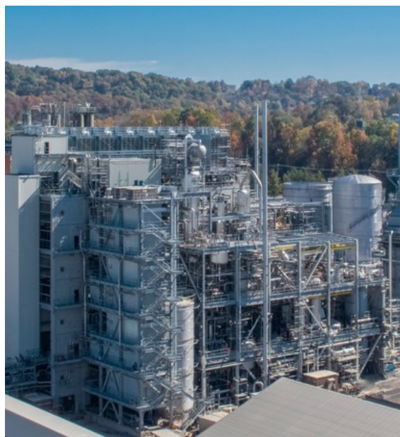
Usine de Kingsport, Tennessee
